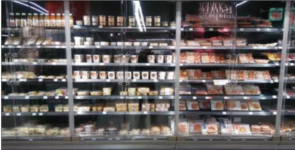
Figure 14.15: Woolworths B packaged foods fridge
