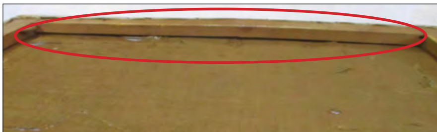
Figure 9: Arched warping of the left vertical stretcher member (photograph by Hannes Elsenbroek)
