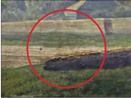
Figure 38: Sigmoid crack on the path connecting with the bridge (photograph by Hannes Elsenbroek)
